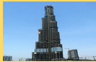
Burj Khalifa, in Dubai, the world's tallest building, shown under construction in 2007 (since completed)
